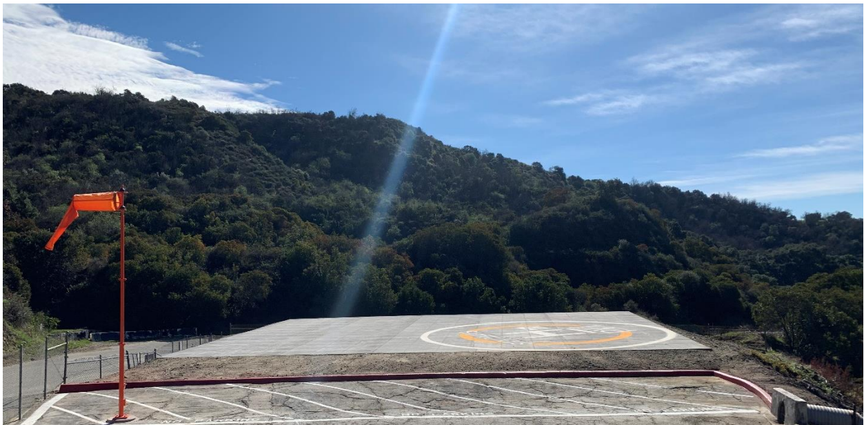
San Dimas Dam – New Heliport
