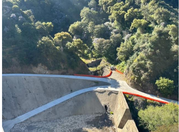
Big Dalton Dam – Access Road
