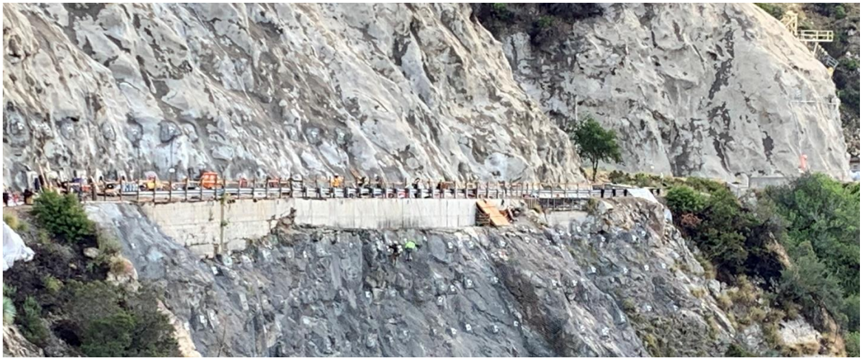
Santa Anita Dam Emergency Access Road Stabilization
