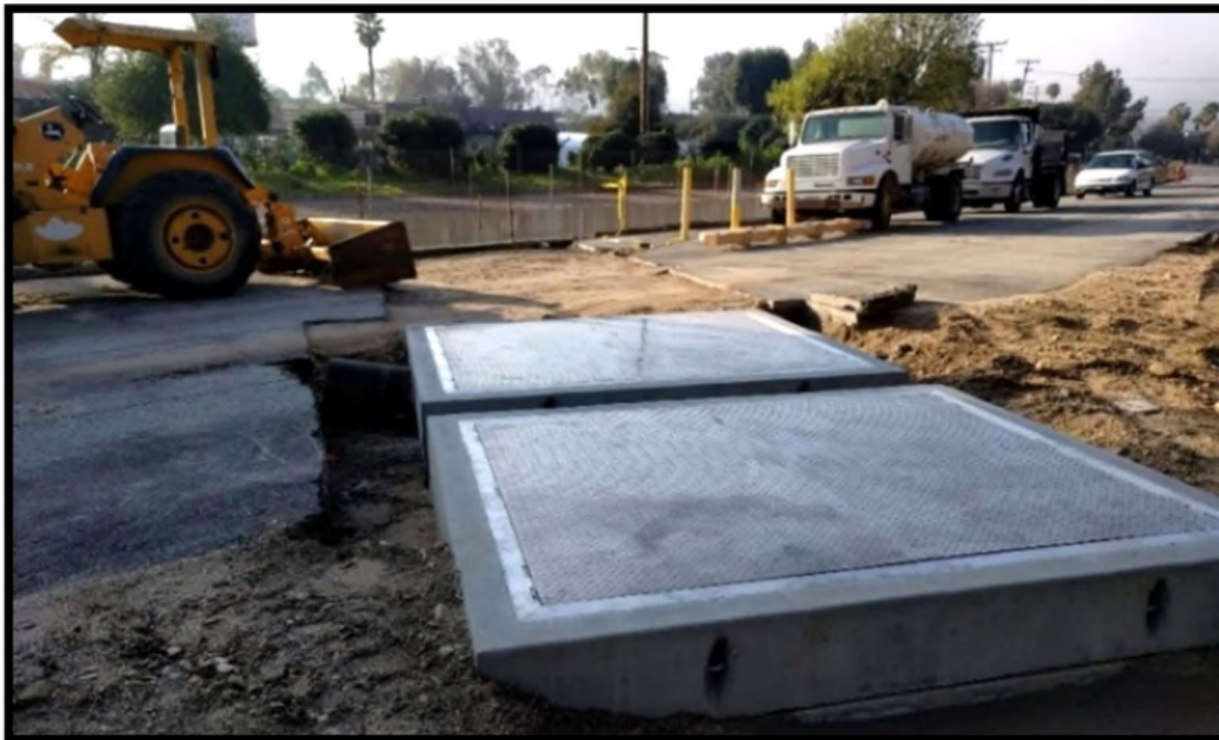
Flow meter vault and diversion box located at the top of the spreading basin.
