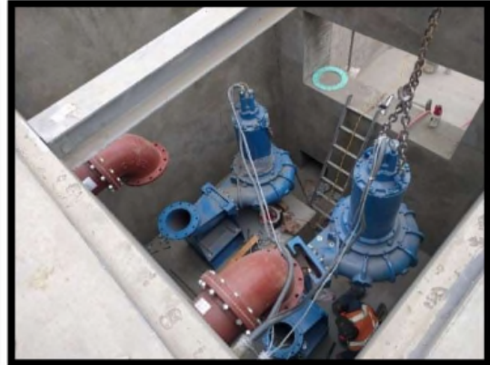
Inside the pump well contains 2 immersible screw impeller pumps, a submersible mixer, a pressure transducer, and a slide gate.
