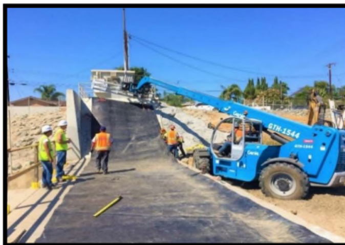
Installation of new rubber dam body onto existing concrete foundation with foundation bolts aligned.
