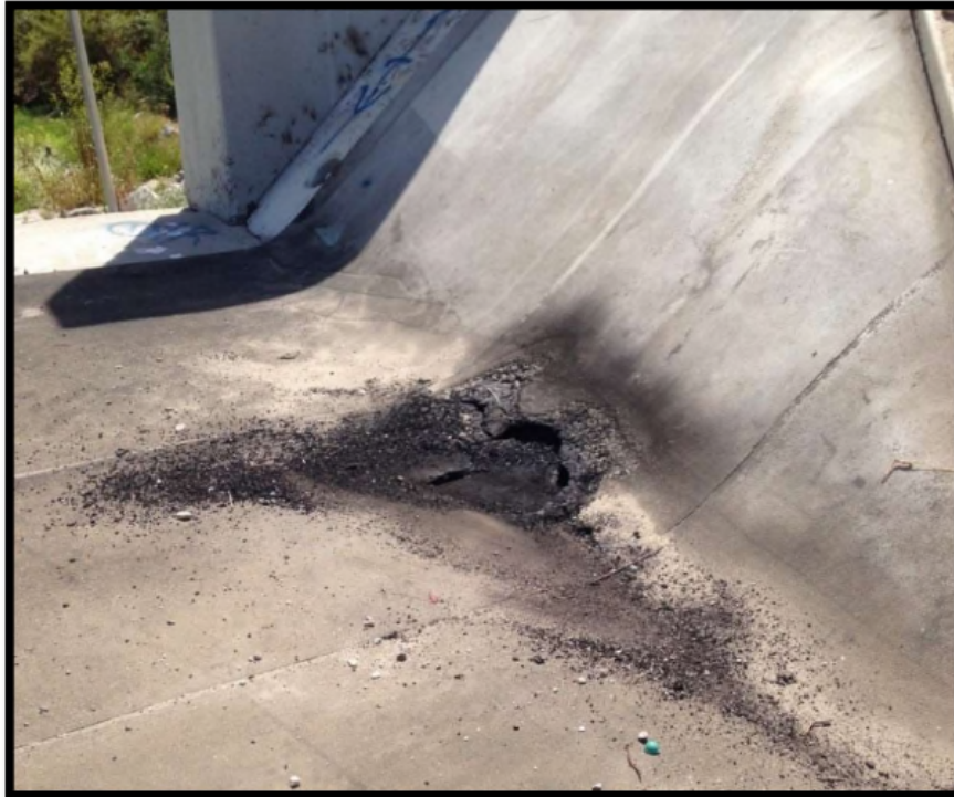
Rubber dam body was damaged and vandalized.
