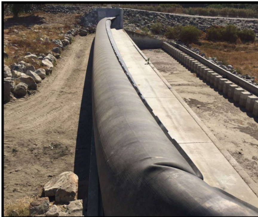
Newly installed and inflated rubber dam.
