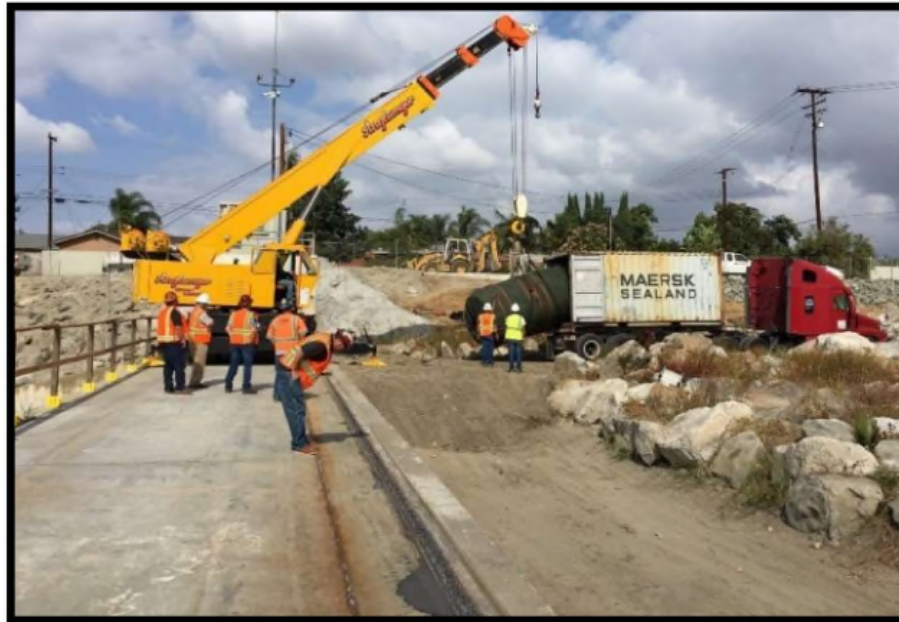
Delivery of the new rolled-up dam body to facility site.
