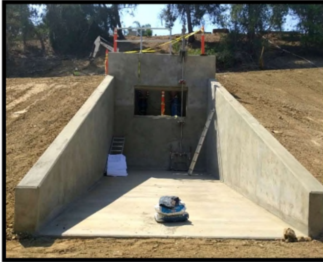
Intake structure at the bottom of the basin.
