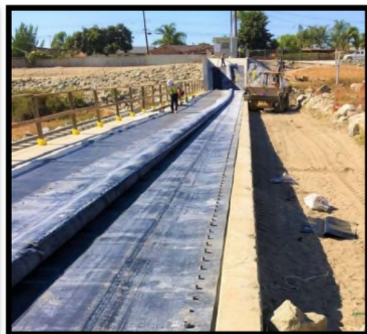
Installation of new rubber dam body onto existing concrete foundation with foundation bolts aligned.
