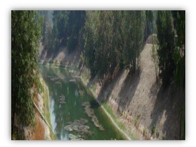
Over the years, fine sediment containing silts and clays have built up in the Spreading Basin, which inhibits groundwater recharge.
